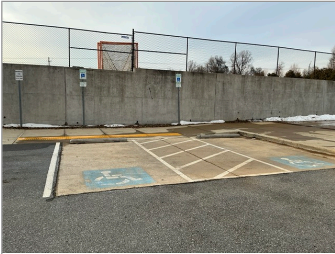
OVERVIEW OF ACCESSIBLE PARKING AREA
