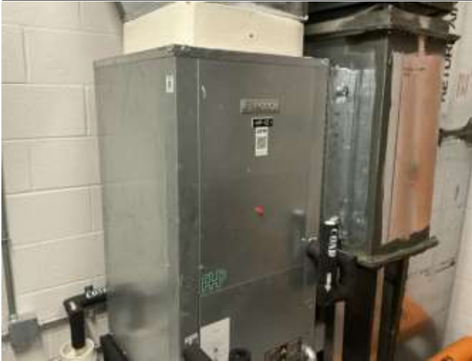
19 - TYPICAL WATER SOURCED HEAT PUMP
