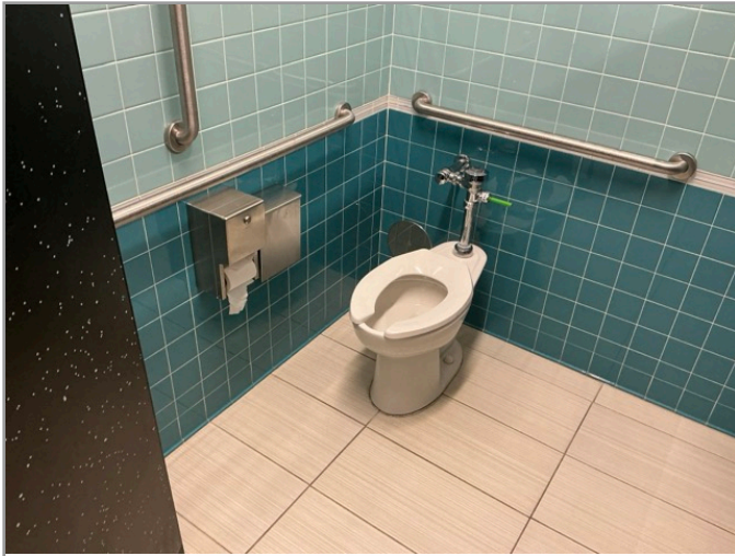
TOILET STALL OVERVIEW
