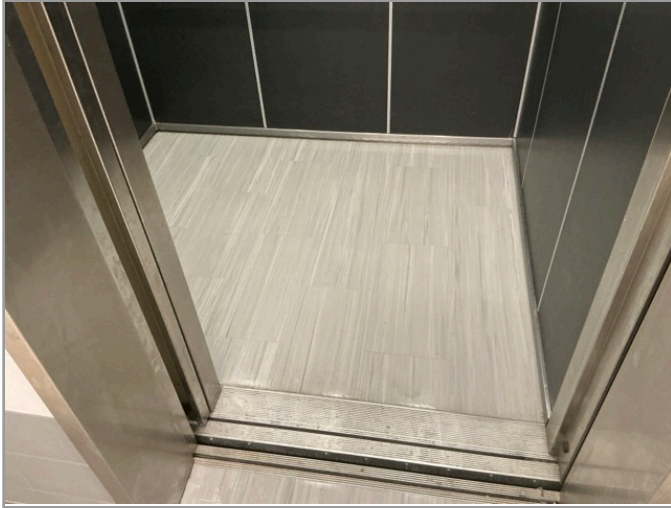
LOBBY LOOKING AT CABS (WITH DOORS OPEN)
